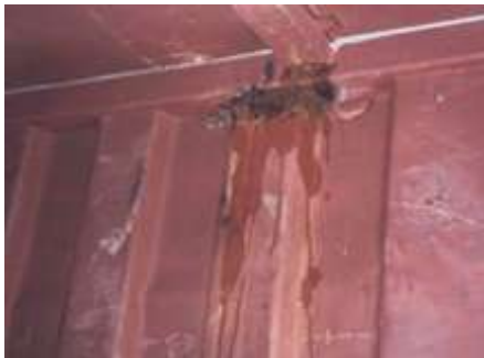
14 Rusted internal roof.
