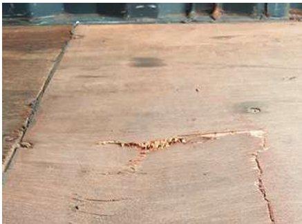
15 Cracked plywood floor. Source: Mētsa Board
