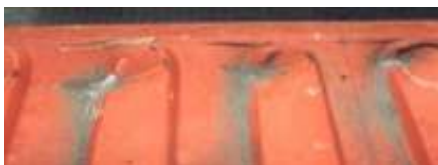
28 Dented external roof.
