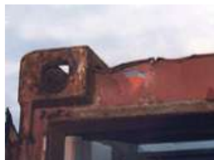
2 Damaged door header.
