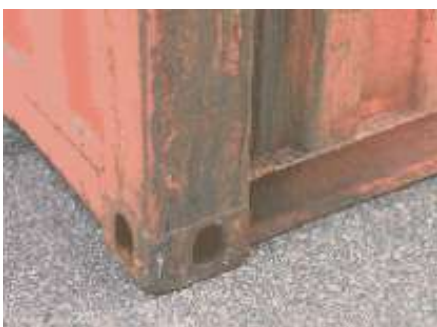
31 Lower corner casting lifting point.
