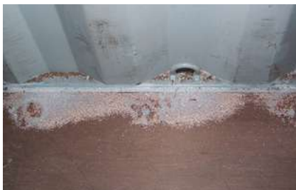
Unacceptable dirty and soiled floor. Source: IF P&C
