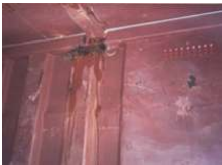
12 Holed internal side panel.
