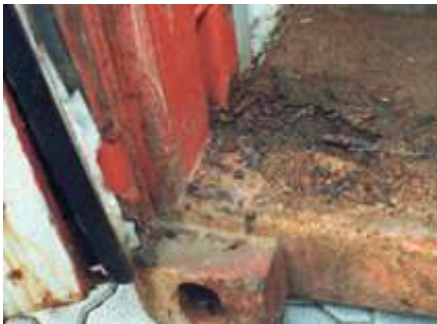
11 Rusted threshold door plate.
